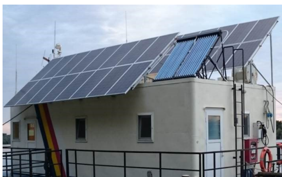
Fig. 16. Mooring pontoon equipped with two types of solar panels
