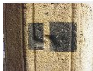
Fig. 4. Laser cleaning on a column from Biserica Doamnei
